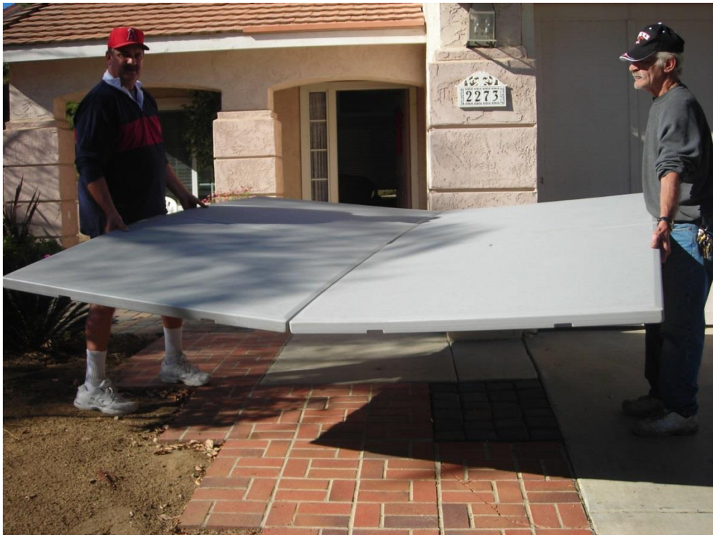
6. Move EZ Pad to spa installation location.
